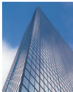
HVAC / Building management
